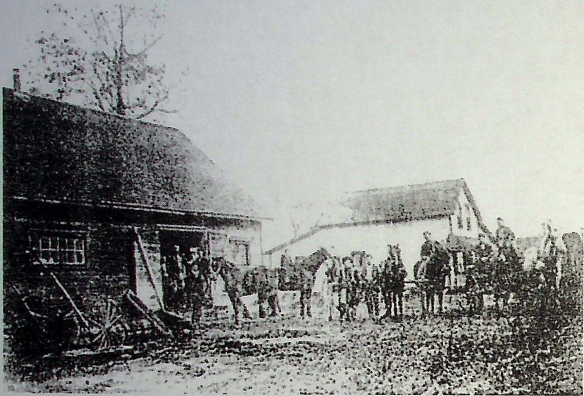
Blacksmith Shop on left, John Armstrong's General Store centre right. courtesy of the Sombra, Ont. Museum.
