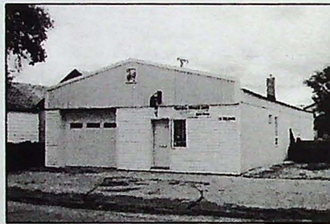
MARANDA'S DEPOT AS IT APPEARS IN 2009 118 MELROSE AVENUE, TRANSCONA
