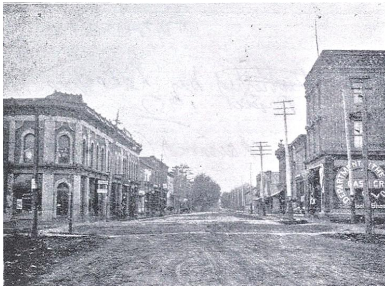
The three storey building to the right was C. A. Quick's store on the N.W. corner of Main and Division Streets in Kingsville.
