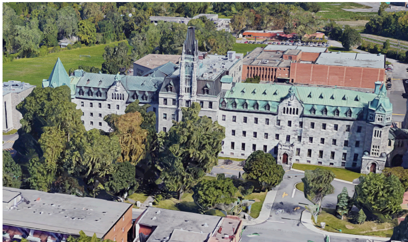
Figure 5. Aerial view of Collège Saint-Laurent as it appears today. Image courtesy of Google Maps.
