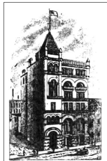
The London and Canadian Loan and Agency at 103 Bay Street West
