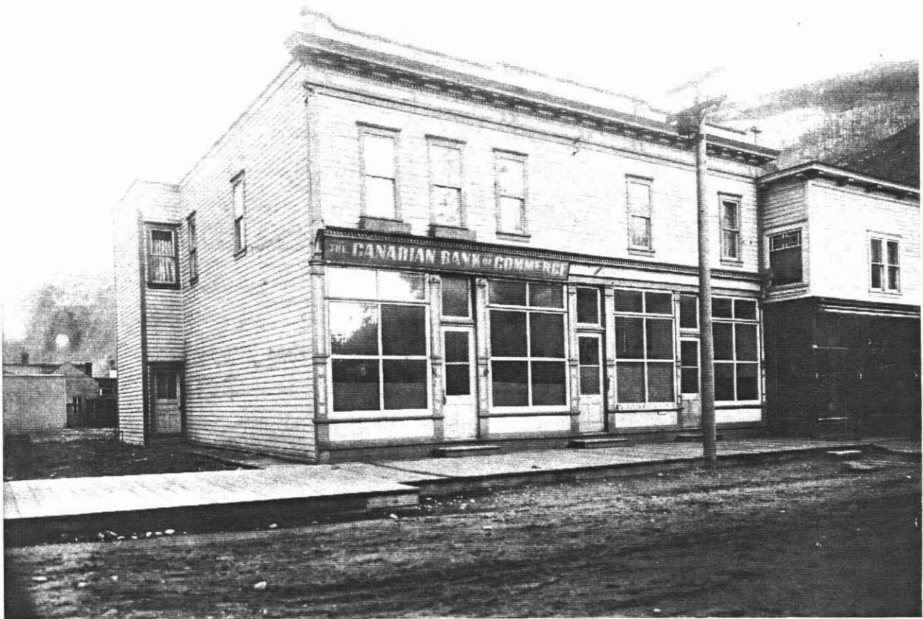
Exterior view of the Skagway branch of The Canadian Bank of Commerce, before the robbery attempt
